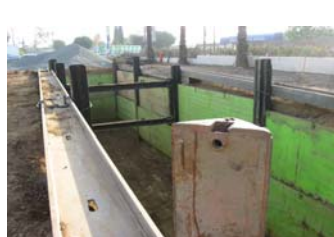
End To End Tank Install
