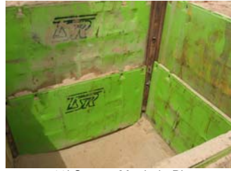
12' Square Manhole Pit
