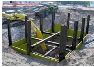
32' X 60' X 24' Deep Soil Remediation
