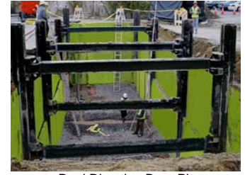
Dual Direction Bore Pit
