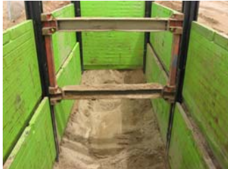
14' X 40' X 16' Deep Bore Pit
