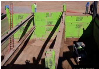
50' X 60' X 16' Deep Triple Tank Install
