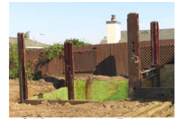
Soil Remediation Next To Homes
